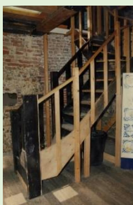
1980's staircase from Old Barge Room to the Great Hall
