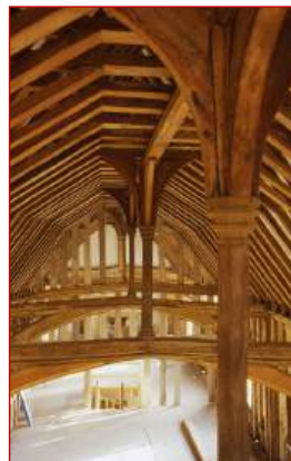
The Great Hall roof
